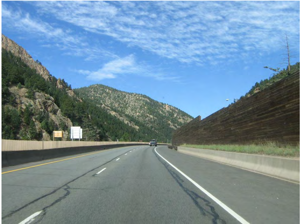
Photo 9. View of I-70 looking west.
