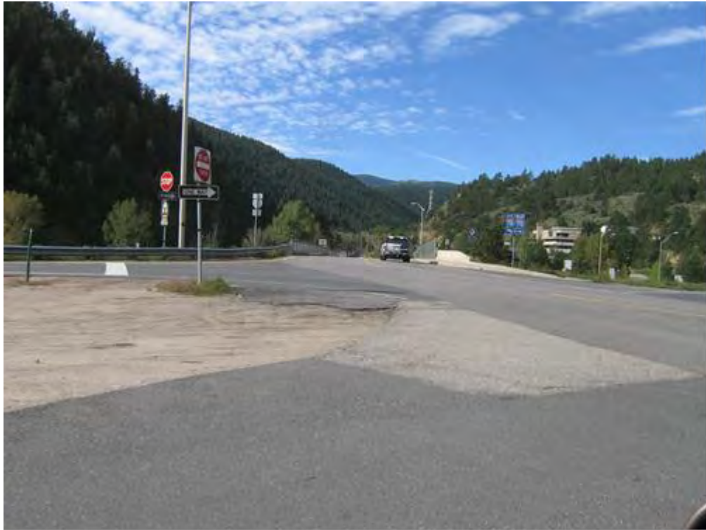
Photo 7. View of structure F-14-E, bridge carrying SH-103 over I-70. Bridge will be replaced during project activities.
