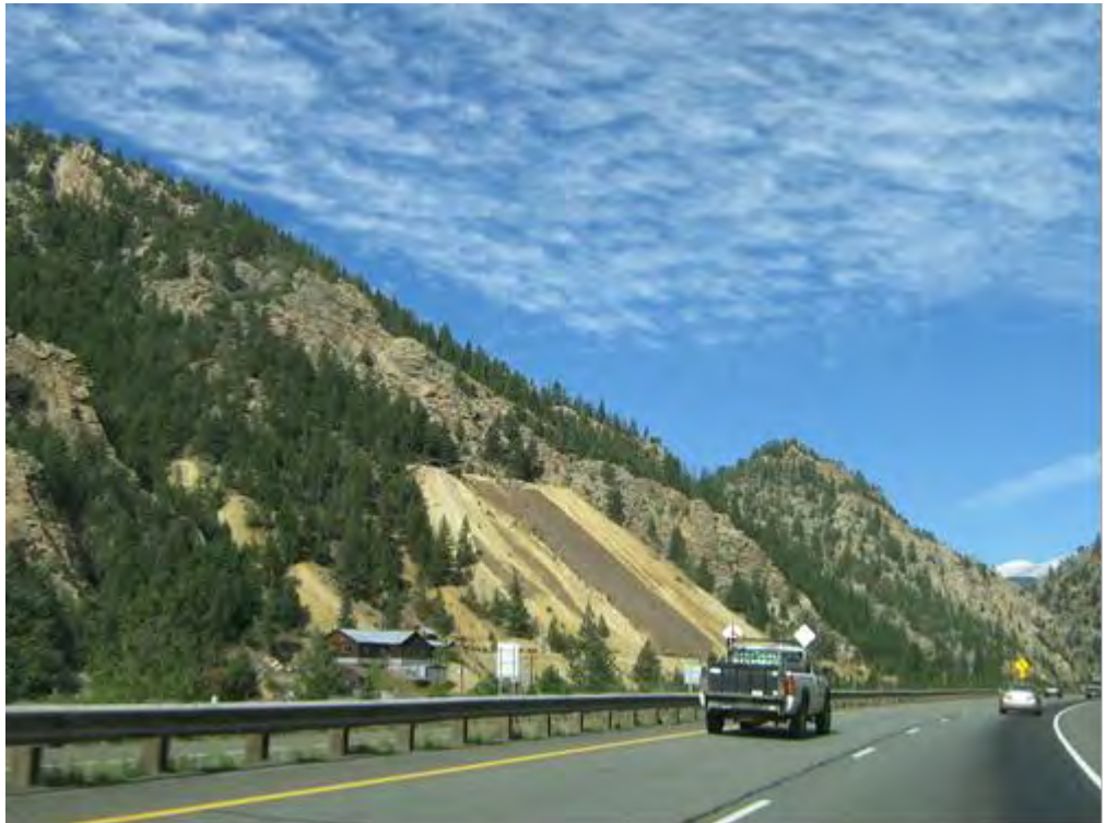
Photo 10. View of the Rockford Mine. Notice the yellow and red discolorations on the slope of the canyon.
